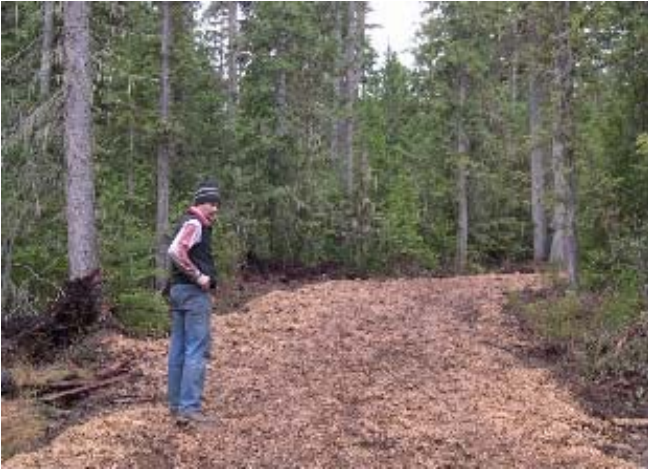
John Thielman On low section of Reino's Run - Woodchip fill Photo: Jeff Lipsett
